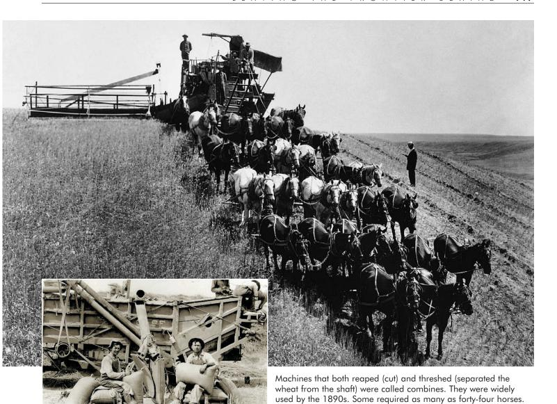
Wheat came down the chute into sacks. A fast worker could sew up to 1,000 sacks per day. Sack sewers in 1911 made \$3 per day.
